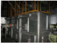
蒸気タービン(右)と発電機(左)<br>
